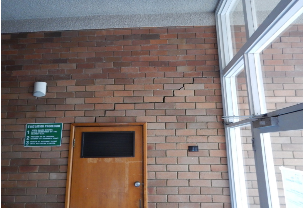
Photo 11 - Cracked wall between main building and Church hall
