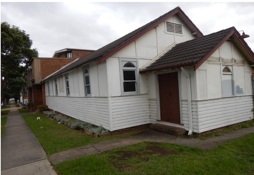
Photo 4 - Possible asbestos building materials on church hall
